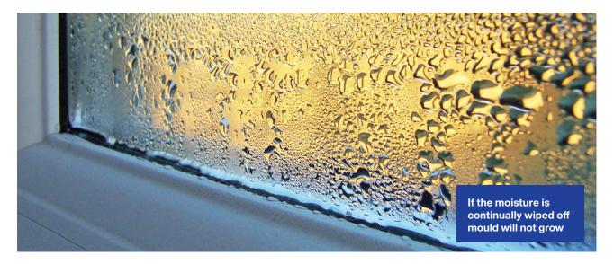
Apartments constructed in the past 15 years have a massive issue with condensation during the cooler months due to inadequate building ventilation.
